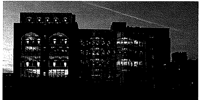
Thomas Jefferson Hall Library, West Point
