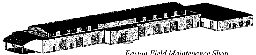
Easton Field Maintenance Shop
