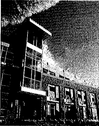
WVU Transportation Center & Garage
