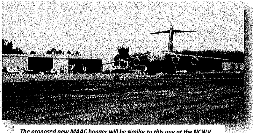
The proposed new MAAC hanger will be similar to this one at the NCWV airport.
