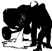
2 DO NOT drain into repair site!
