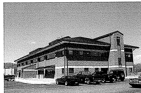
WVDOH D-6 Office Building, Moundsville, WV
