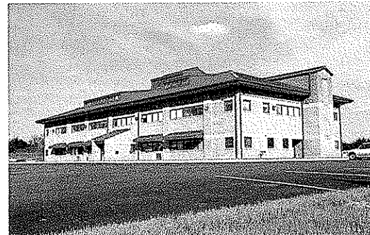
WVDOH D-10 Office Building, Gardner, WV
