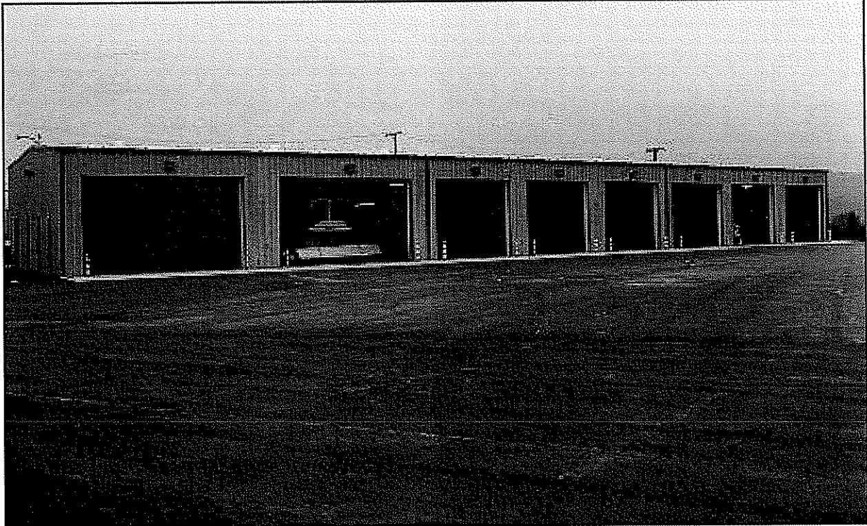
The 7 bay facility was Chapman Technical Group's first project for Yeager Airport.
