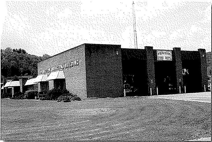
Princeton Municipal Building & Fire Department
