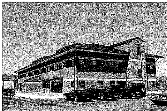
WVDOH D-6 Office Building, Moundsville, WV
