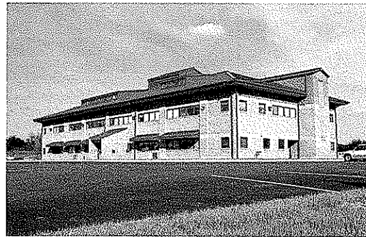
WVDOH D-10 Office Building, Gardner, WV
