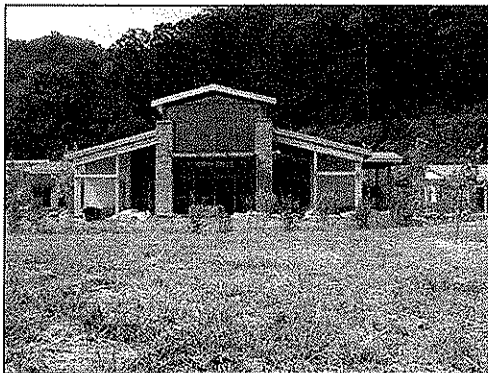
Sandstone Visitor/Orientation Center. The project site is located in a remote section of West Virginia, with few public utilities available as energy sources for the project
