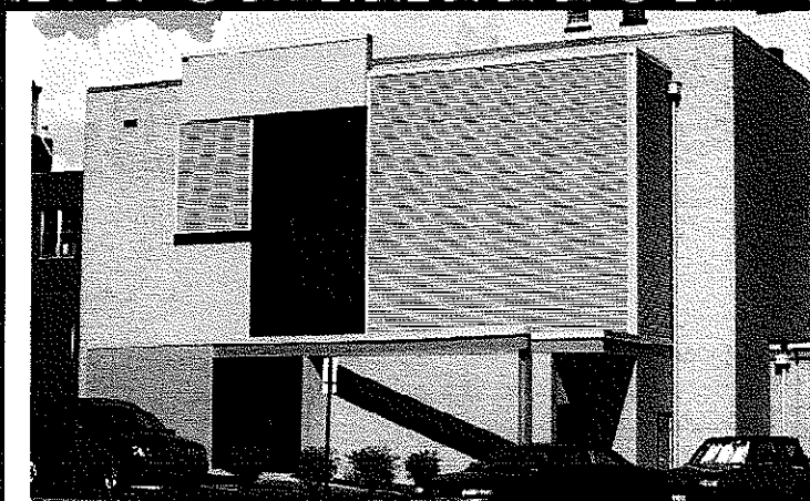
Dr. Ganzer Office Building
