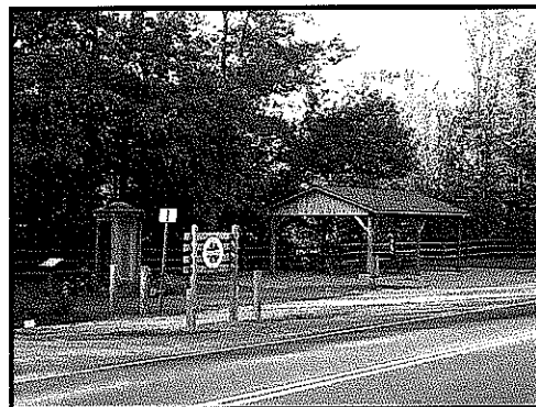
City of Shinnston, WV Rails to Trails Trailhead
