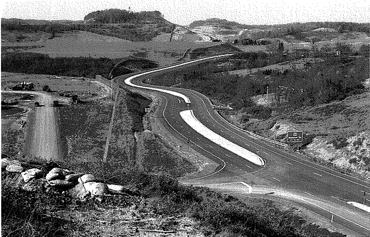
ROUTE 279, NORTH BRIDGEPORT BYPASS – COMPLETED IN 2000
