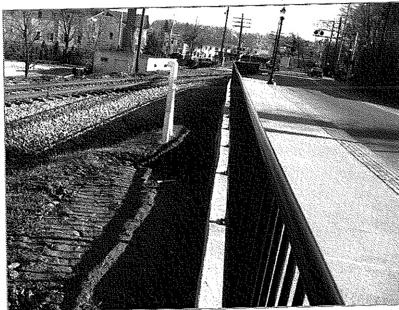
Safety Rail Along North Side of Main Street
