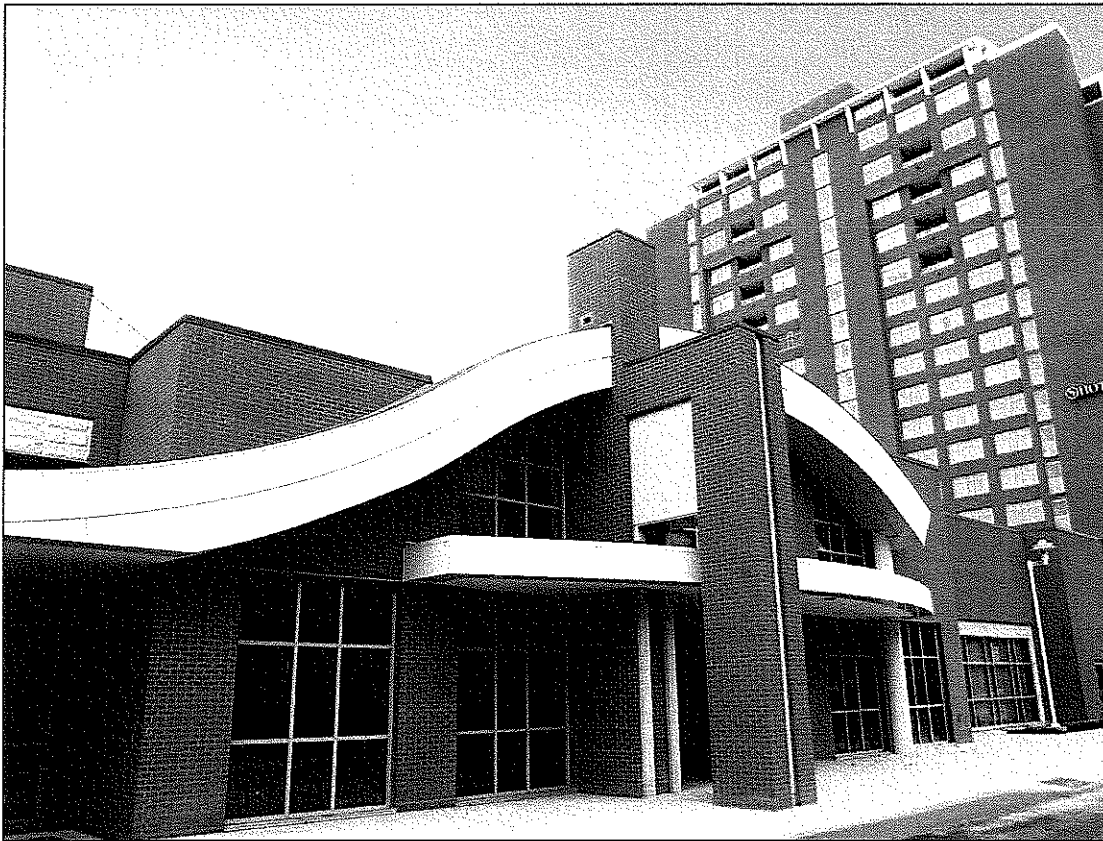
(Currently Under Construction)
