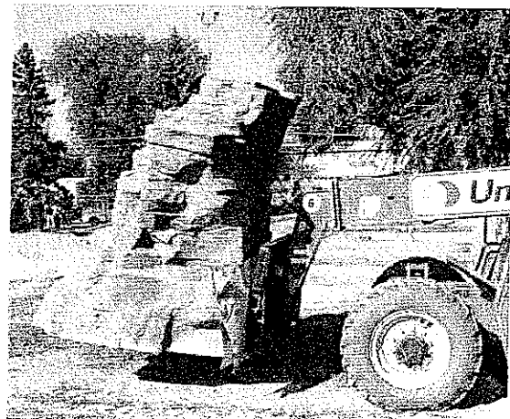
Lower the King Peak into place with a Lull-type Forklift, Crane or Boom
