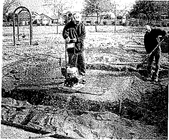
Start with a base of compacted aggregate
