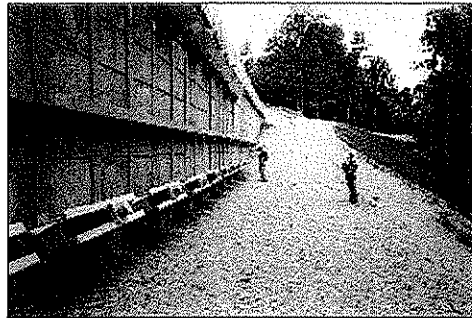
Finished wall with anchors
