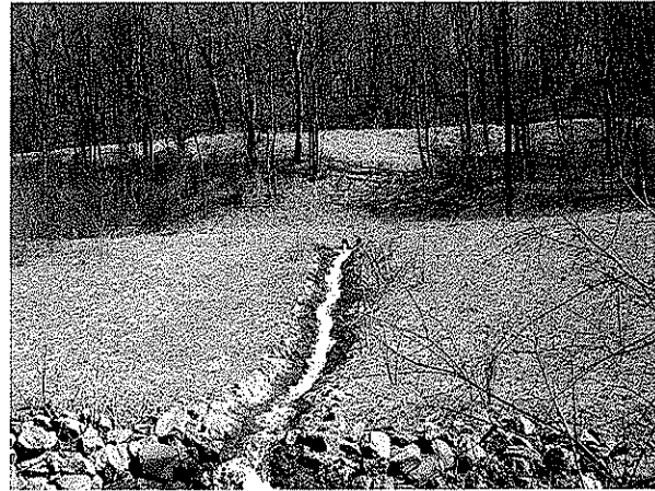
Wet mine seal with rip rap channel
