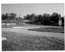
project consisted of The 700 of approximately tons asphalt base course, 350 tons of asphalt wearing course, crushed aggregate base course, drop inlet risers and existing concrete removal sidewalk installation of handicap ramps. G&O is responsible for the
