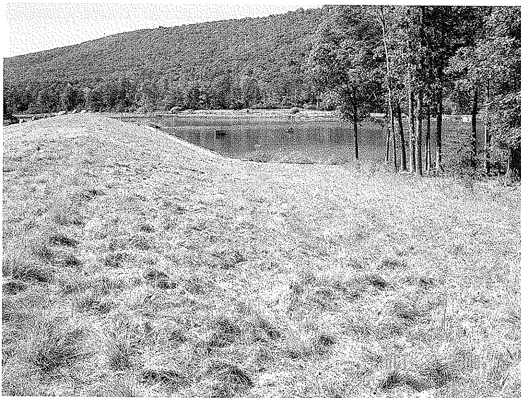
WARDEN LAKE DAM MODIFICATION, HARDY CO., WV
