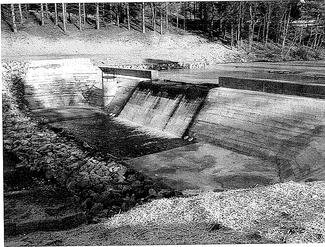
THOMAS DAM MODIFICATION, THOMAS, WV
