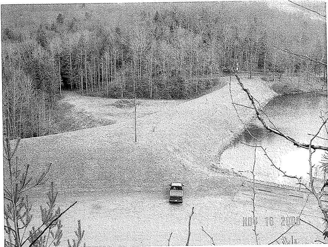
PLUM ORCHARD DAM MODIFICATION, FAYETTE CO., WV
