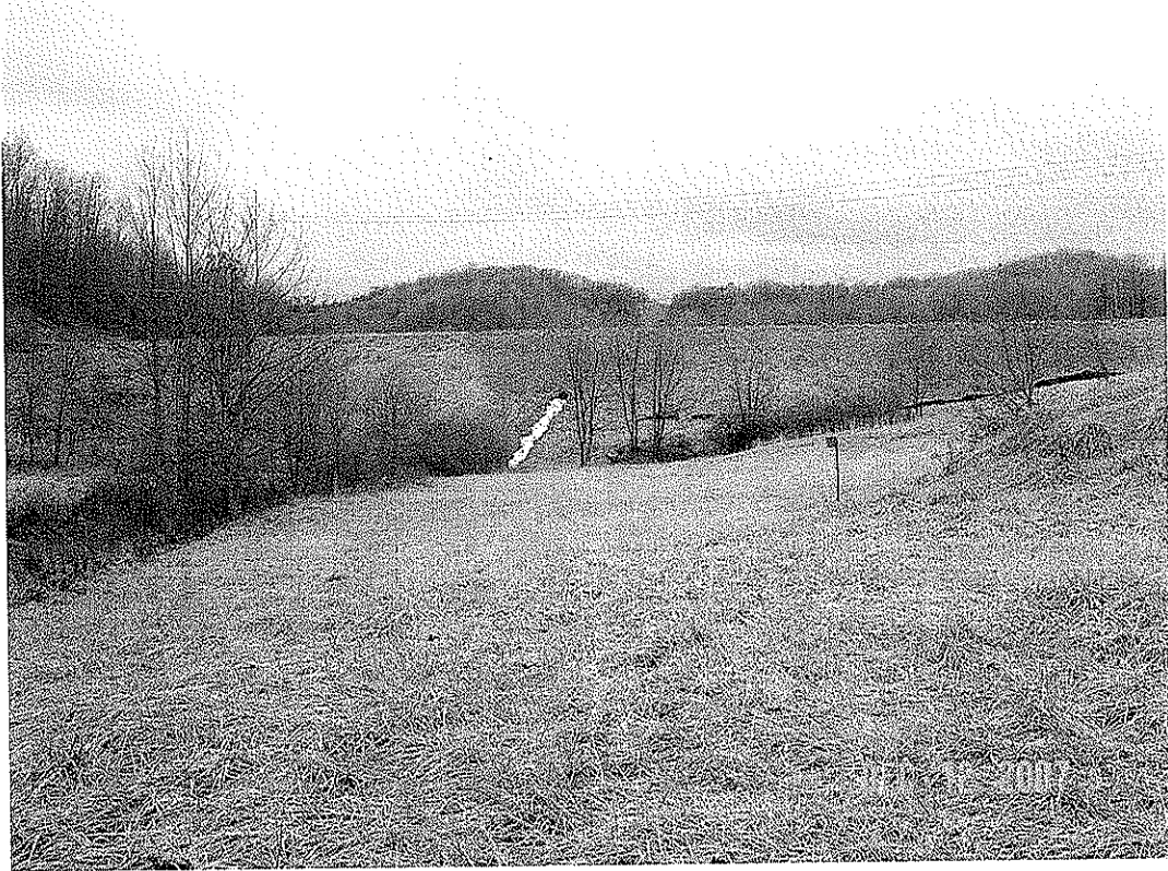
LEMLEY DAM MODIFICATION, MONONGALIA CO., WV
