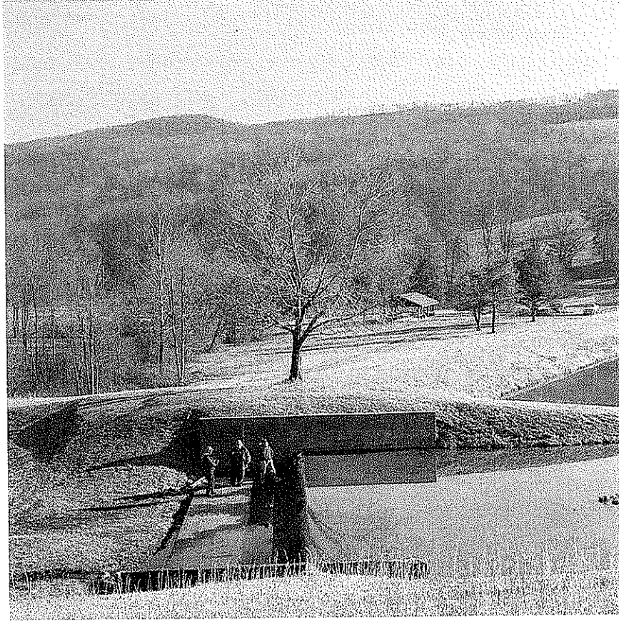
BELINGTON DAM MODIFICATION, BELINGTON, WV
