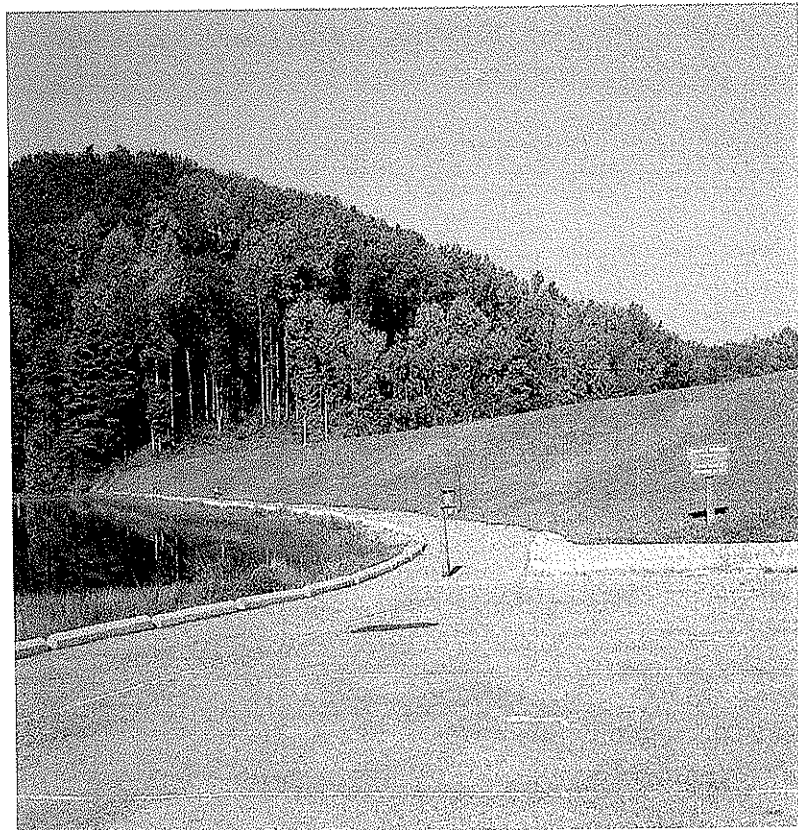
TETER CREEK DAM MODIFICATION, BARBOUR CO., WV
