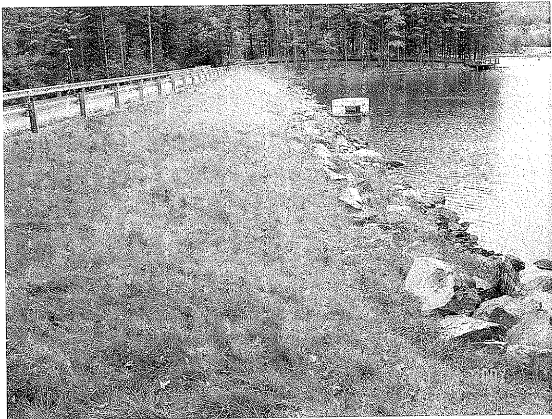
MONCOVE DAM MODIFICATION, MONROE CO., WV
