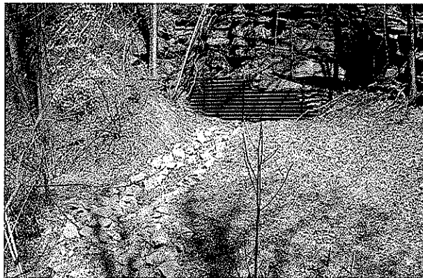
Bat Gate with rip rap channel
