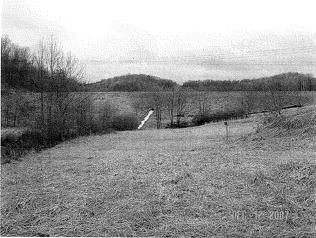
LEMLEY DAM MODIFICATION, MONONGALIA CO., WV
