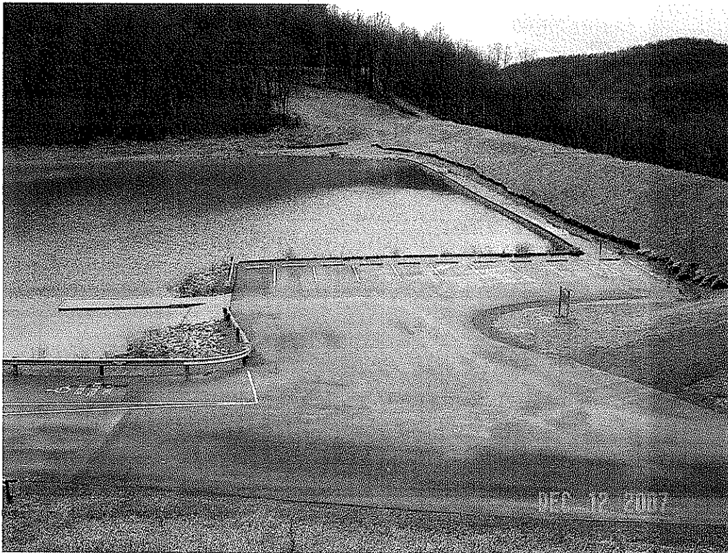
BAILEY DAM MODIFICATION, MONONGALIA CO., WV
