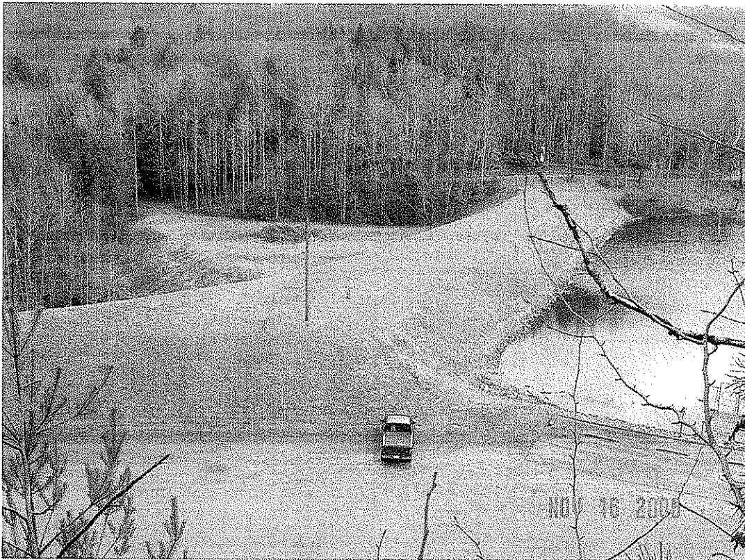
PLUM ORCHARD DAM MODIFICATION, FAYETTE CO., WV
