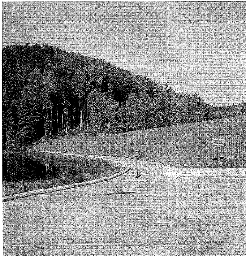
TETER CREEK DAM MODIFICATION, BARBOUR CO., WV
