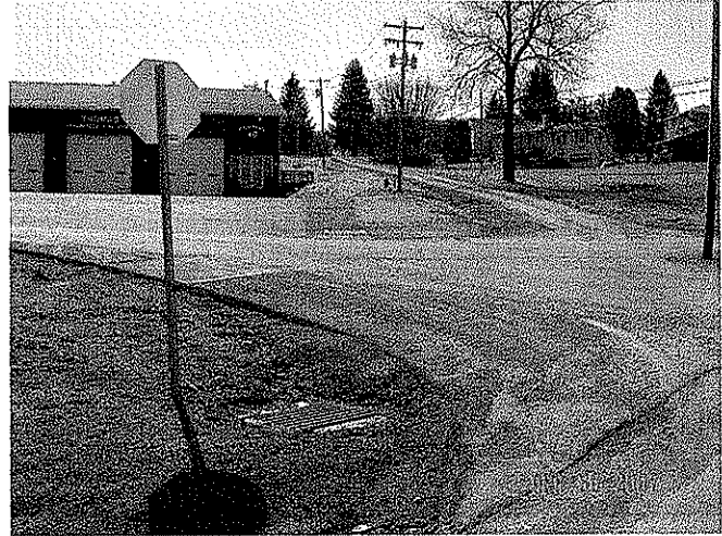
New Storm Drains and Catch Basins
