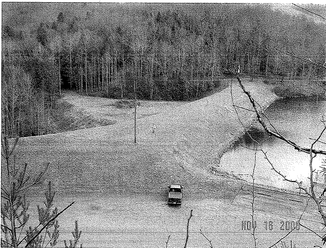
PLUM ORCHARD DAM MODIFICATION, FAYETTE CO., WV
