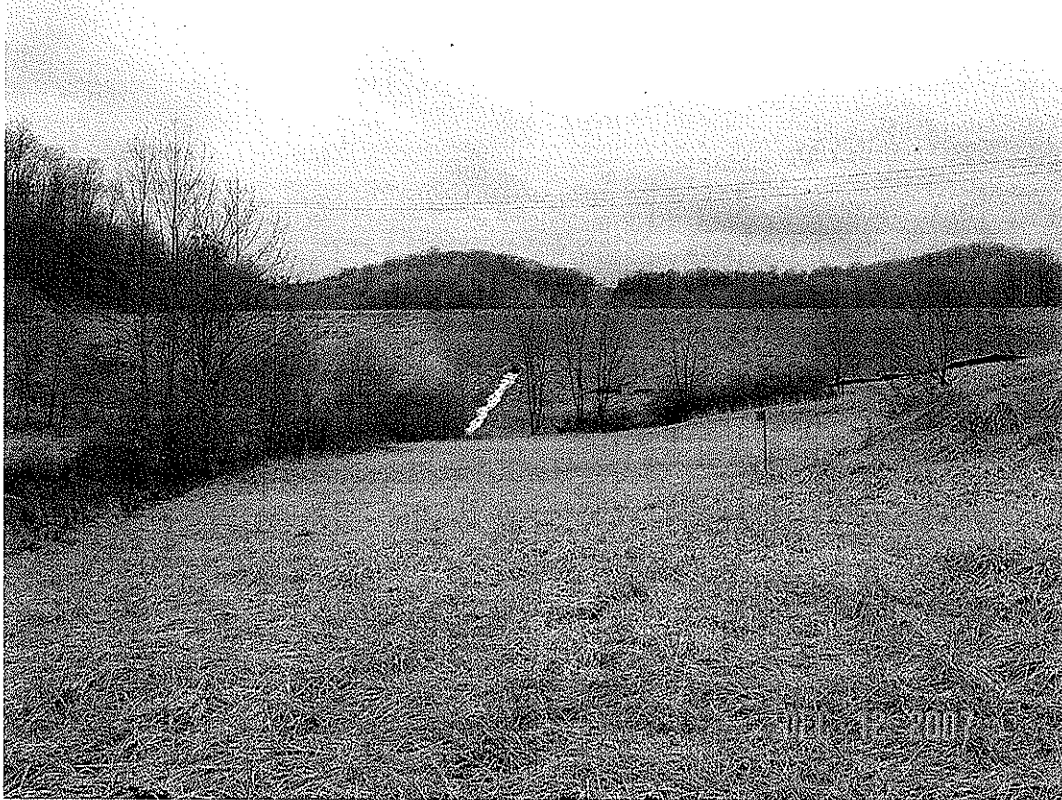
LEMLEY DAM MODIFICATION, MONONGALIA CO., WV
