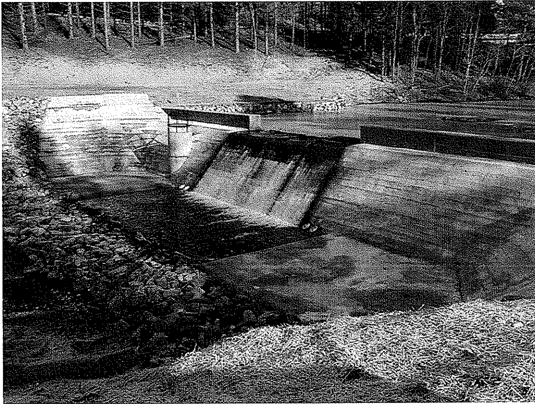
THOMAS DAM MODIFICATION, THOMAS, WV
