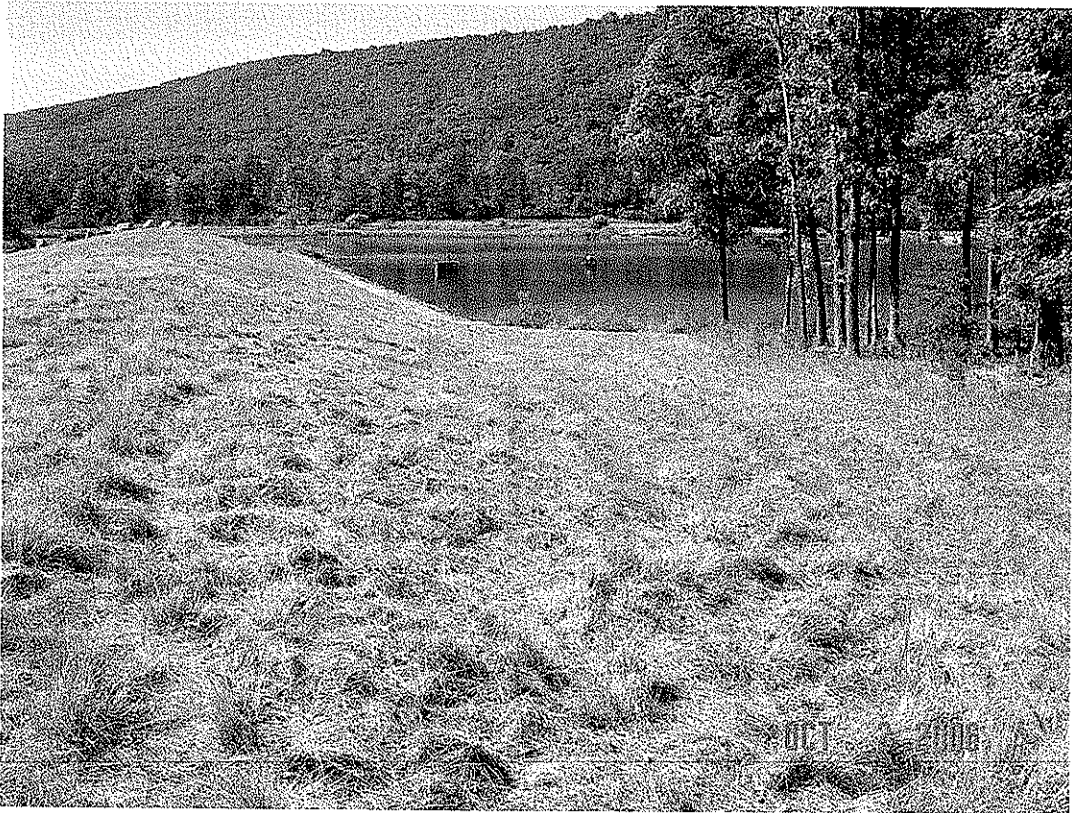
WARDEN LAKE DAM MODIFICATION, HARDY CO., WV
