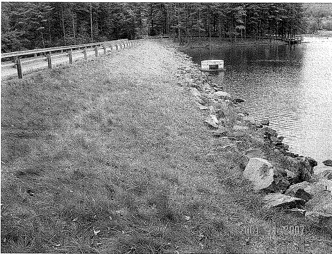
MONCOVE DAM MODIFICATION, MONROE CO., WV
