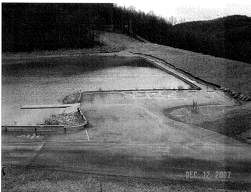
BAILEY DAM MODIFICATION, MONONGALIA CO., WV
