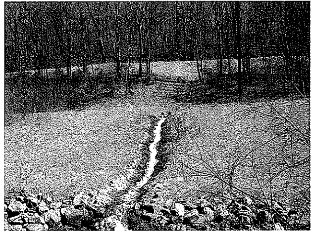
Wet mine seal with rip rap channel
