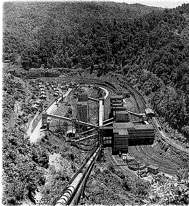
Picture 1 is a circa 1950's image of the working prep plant at Gary, WV.
