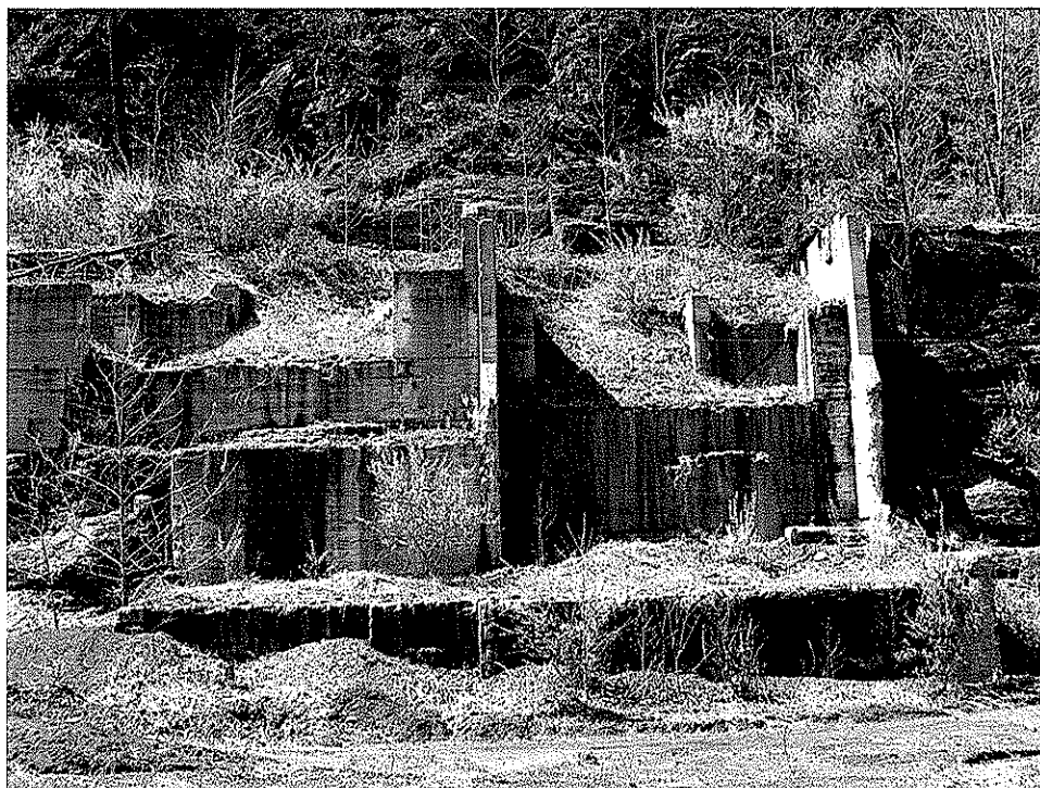
Picture 5 shows reinforced concrete ruins of the prep plant.
