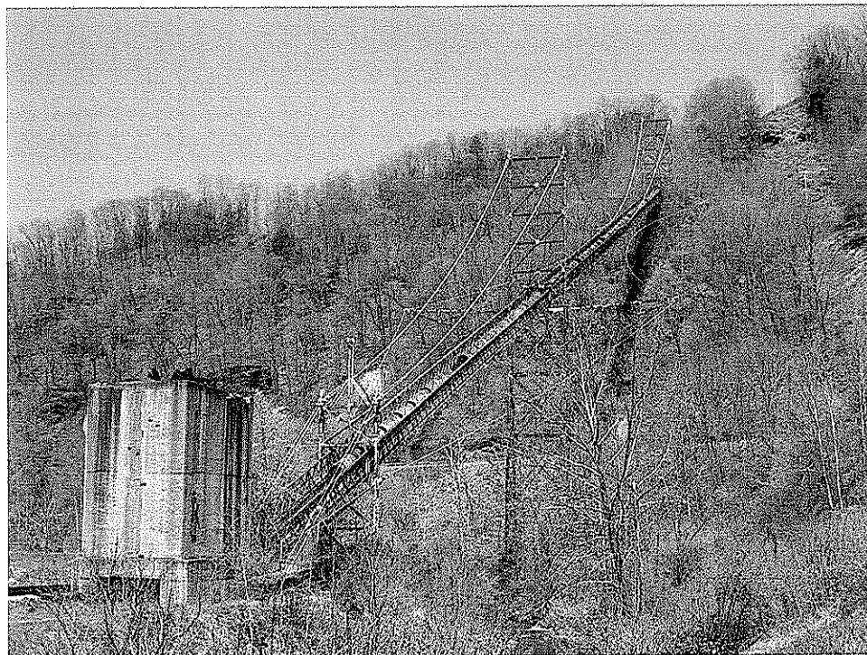
Picture 2 shows the remains of the prep plant conveyor belt.
