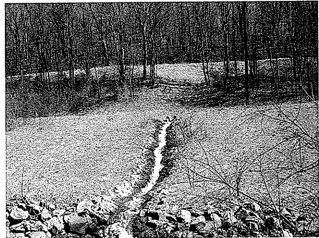
Wet mine seal with rip rap channel
