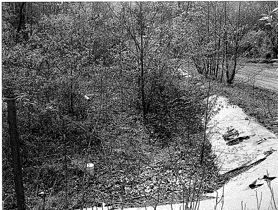
Picture 7 shows an abandoned filtration pond.
