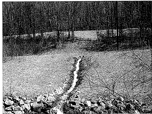
Wet mine seal with rip rap channel
