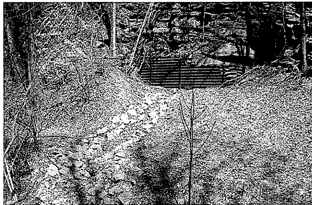
Bat Gate with rip rap channel
