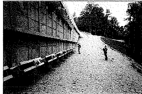
Finished wall with anchors
