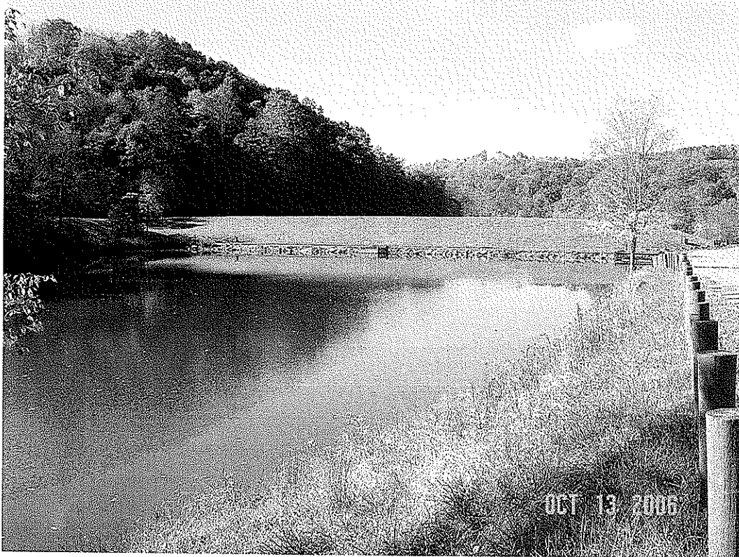
JIMMY LEWIS DAM MODIFICATION, MERCER CO., WV
