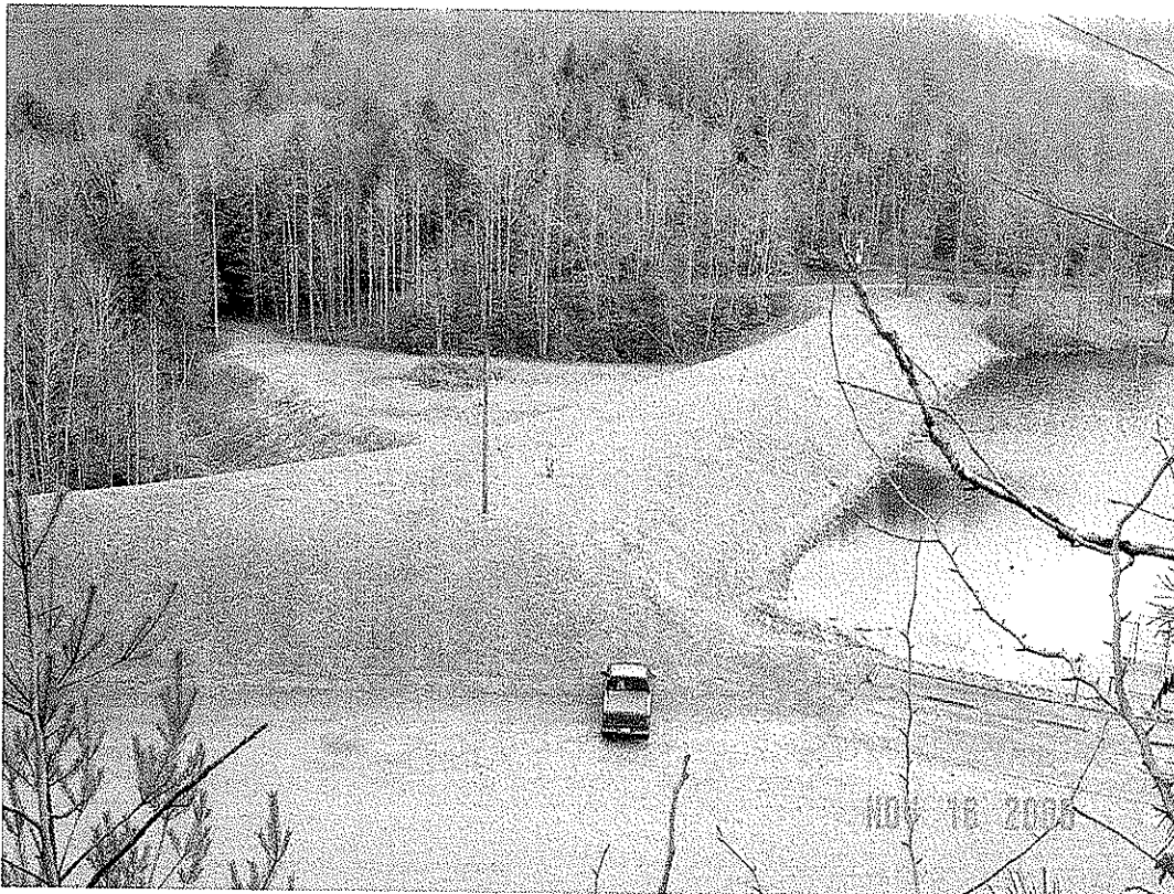
PLUM ORCHARD DAM MODIFICATION, FAYETTE CO., WV
