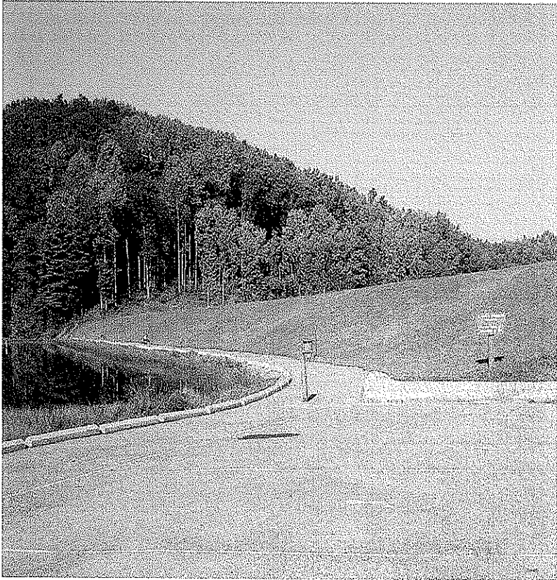
TETER CREEK DAM MODIFICATION, BARBOUR CO., WV
