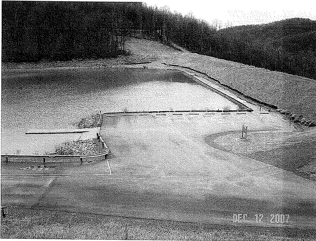
BAILEY DAM MODIFICATION, MONONGALIA CO., WV
