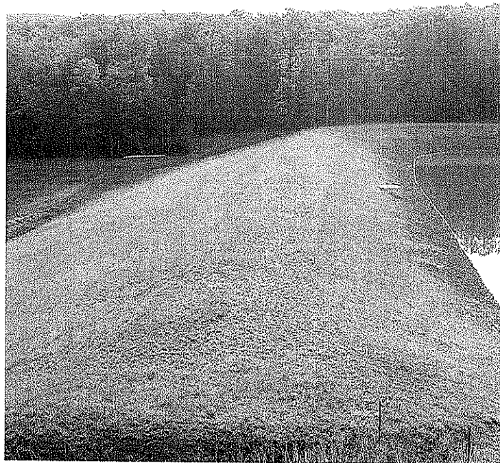
WILSON DAM MODIFICATION, HAMPSHIRE CO., WV
