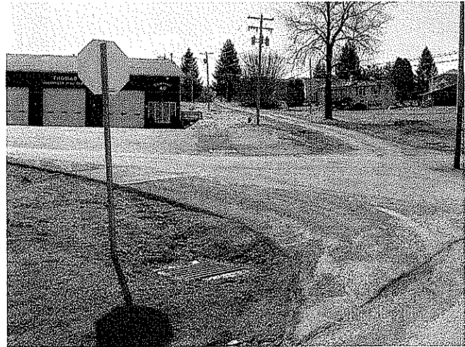
New Storm Drains and Catch Basins
