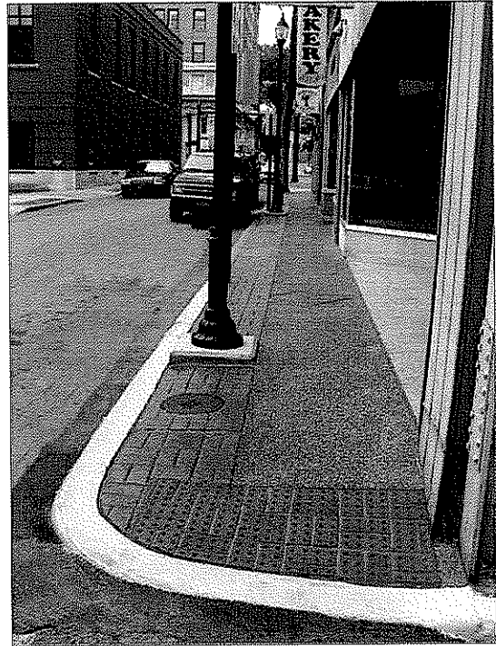
West Side of South Third Street
