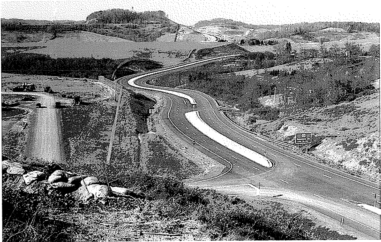
ROUTE 279, NORTH BRIDGEPORT BYPASS – COMPLETED IN 2000
