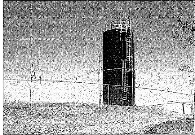
43,000 Gallon Salem Ridge Water Storage Tank
