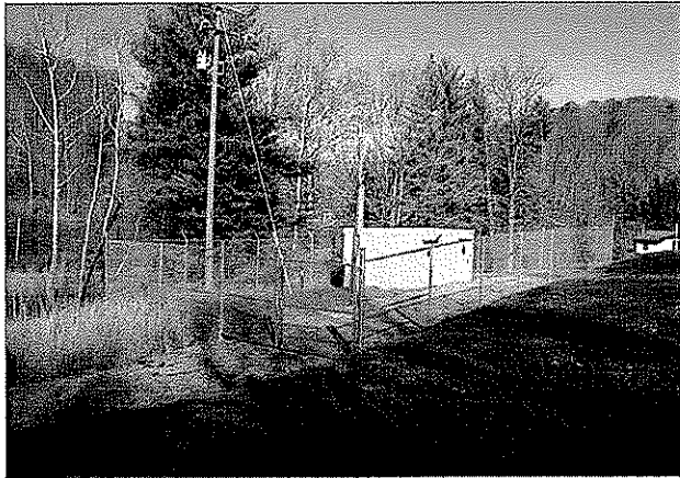
50 GPM Wilsontown Booster Station
