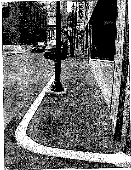
West Side of South Third Street
