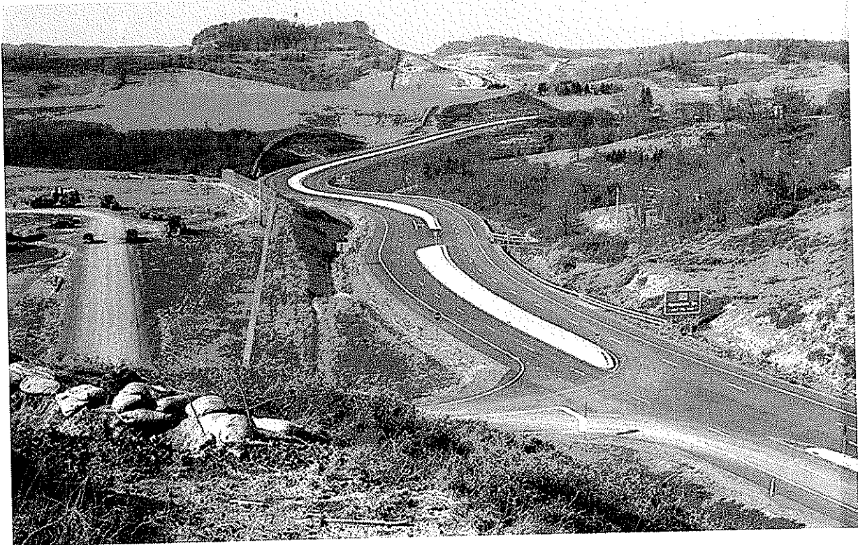
ROUTE 279, NORTH BRIDGEPORT BYPASS - COMPLETED IN 2000
