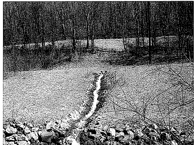
Wet mine seal with rip rap channel
