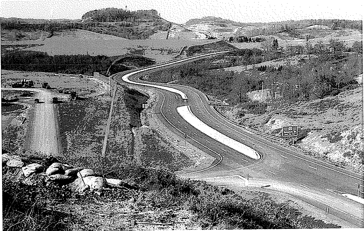
ROUTE 279, NORTH BRIDGEPORT BYPASS - COMPLETED IN 2000
