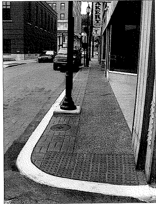
West Side of South Third Street
