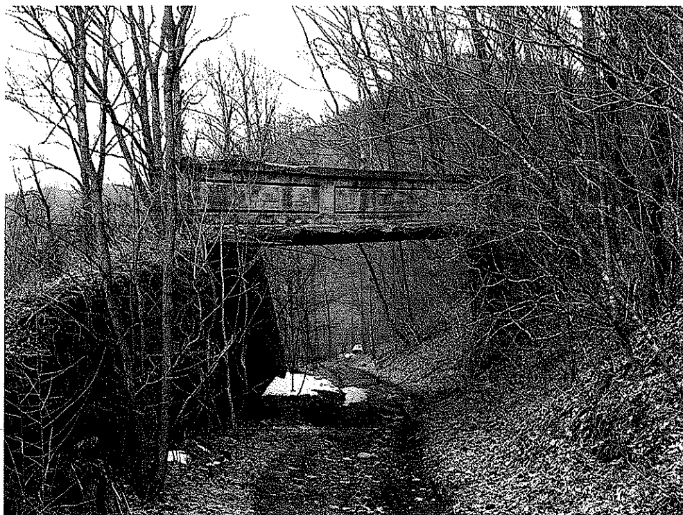
Picture 5 shows an old overpass.
