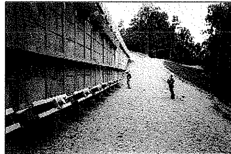
Finished wall with anchors
