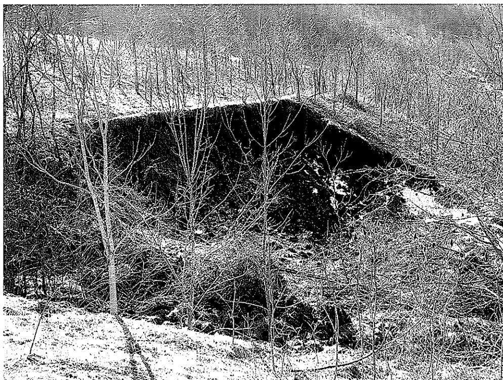
Picture 1 is of an eroded area of the refuse pile.
