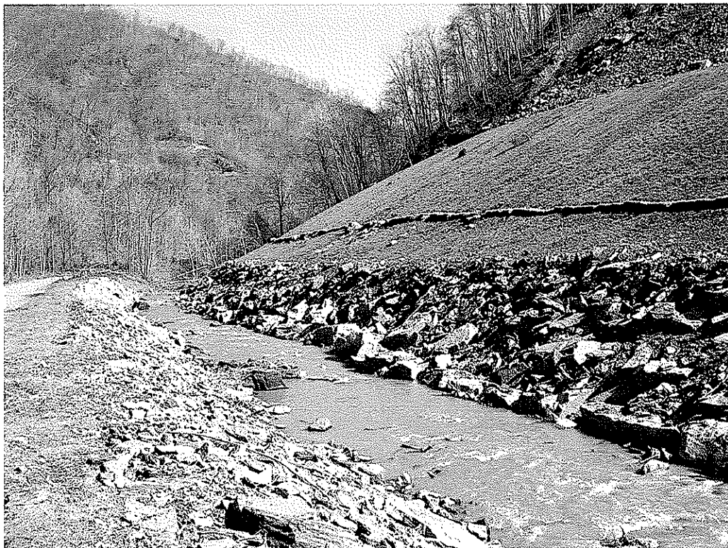
Picture 7 shows stream stabilization on another section of Hazy Creek.
