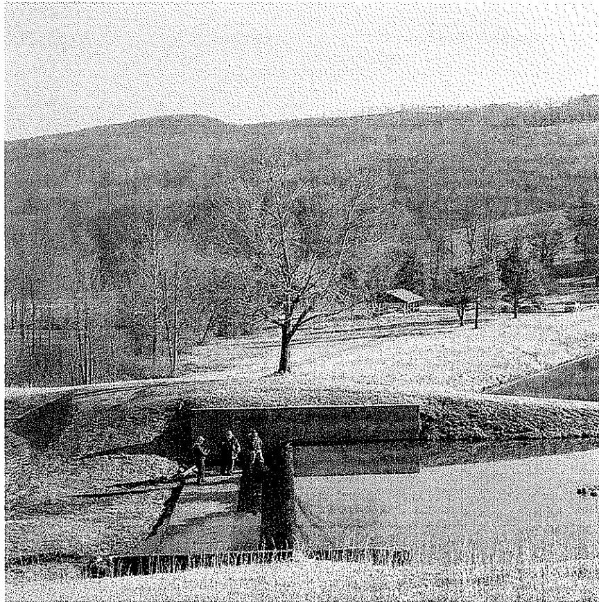
BELINGTON DAM MODIFICATION, BELINGTON, WV
