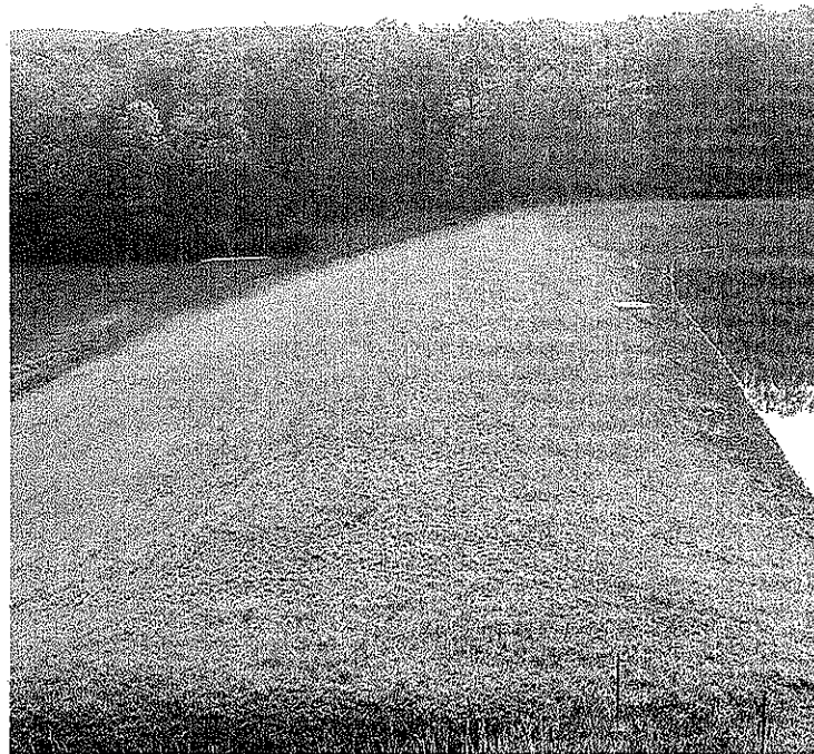
WILSON DAM MODIFICATION, HAMPSHIRE CO., WV
