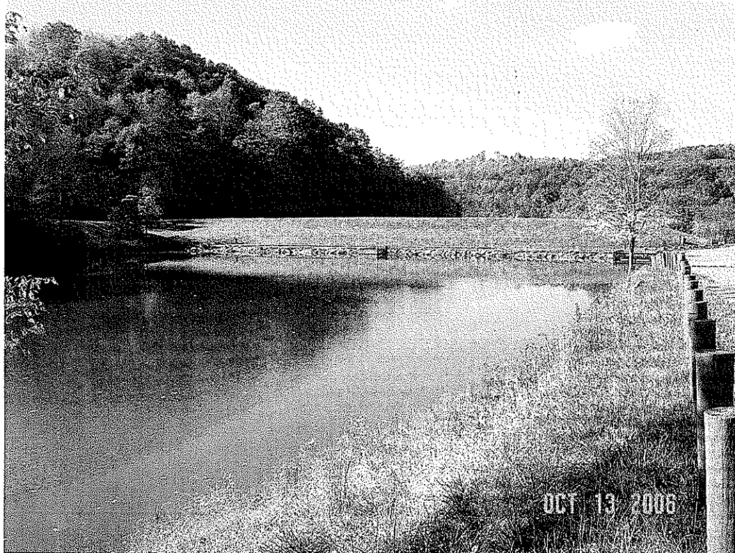
JIMMY LEWIS DAM MODIFICATION, MERCER CO., WV
