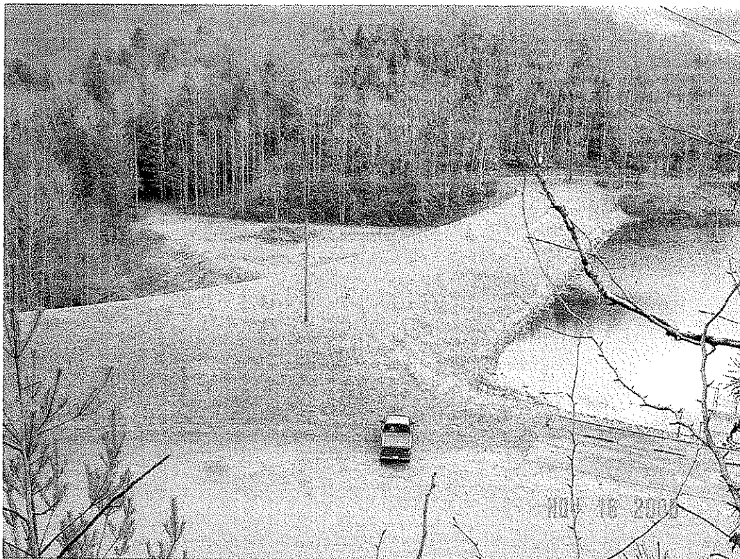
PLUM ORCHARD DAM MODIFICATION, FAYETTE CO., WV
