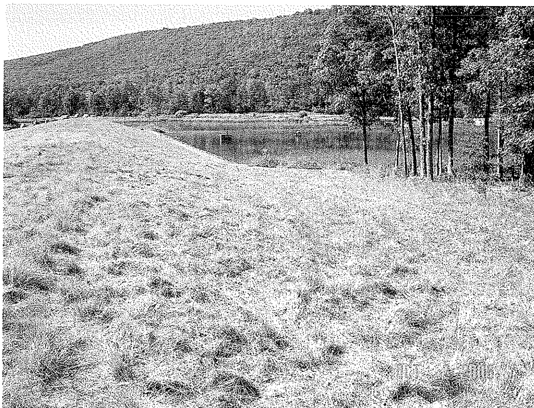
WARDEN LAKE DAM MODIFICATION, HARDY CO., WV
