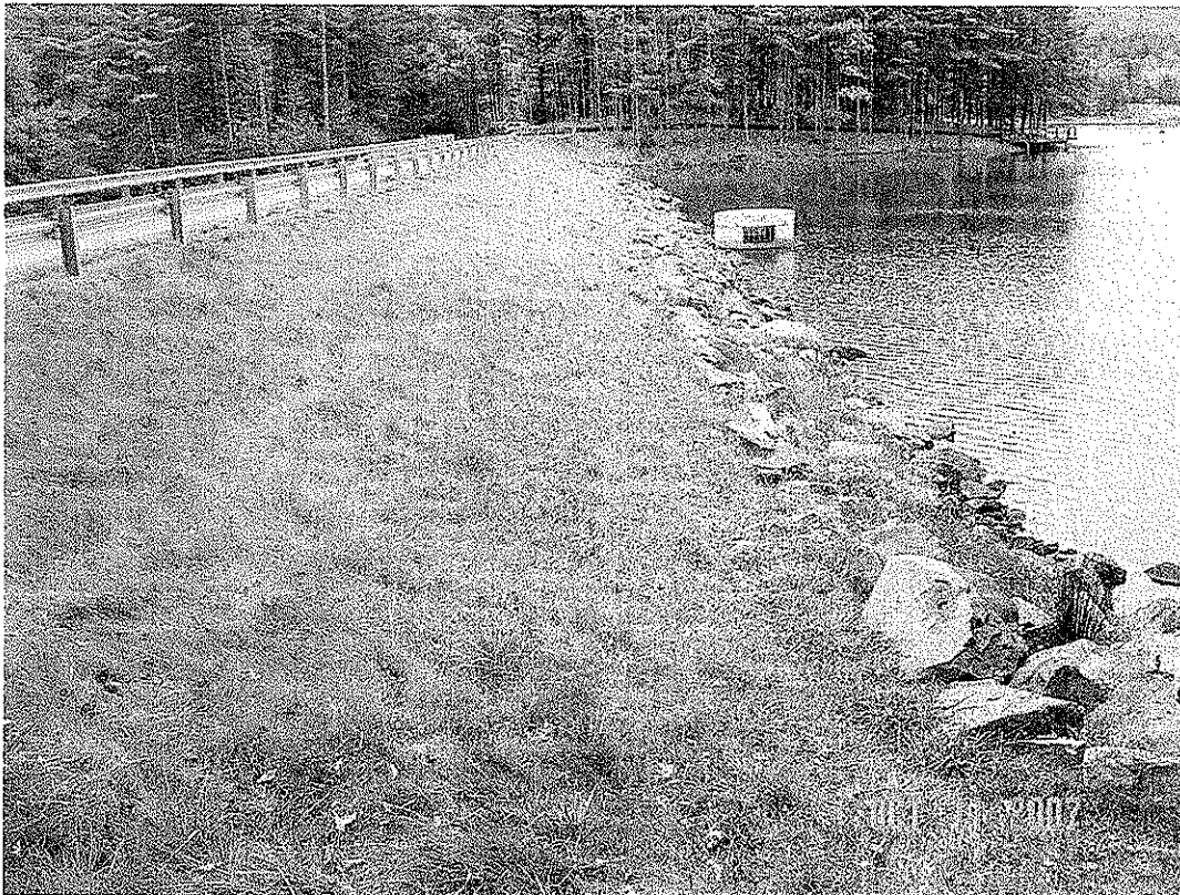
MONCOVE DAM MODIFICATION, MONROE CO., WV
