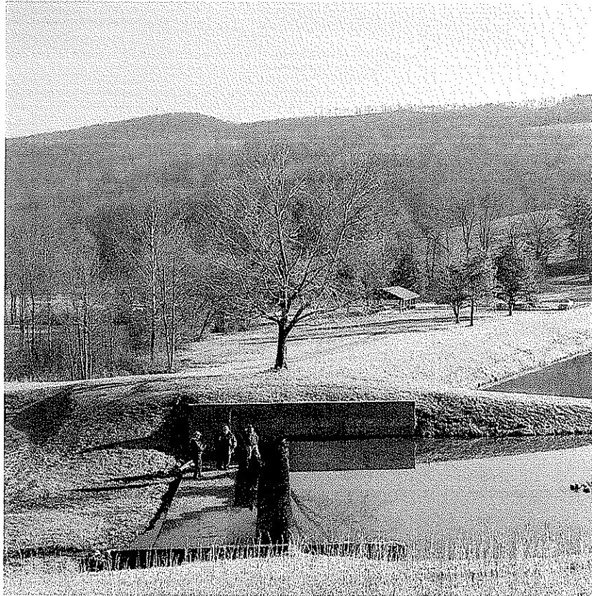
BELINGTON DAM MODIFICATION, BELINGTON, WV
