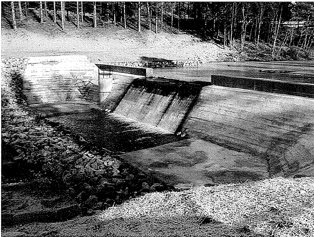
THOMAS DAM MODIFICATION, THOMAS, WV
