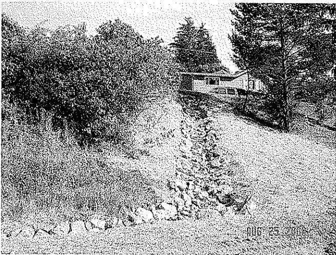
Erosion Repair – Rip Rap Armored Ditch
