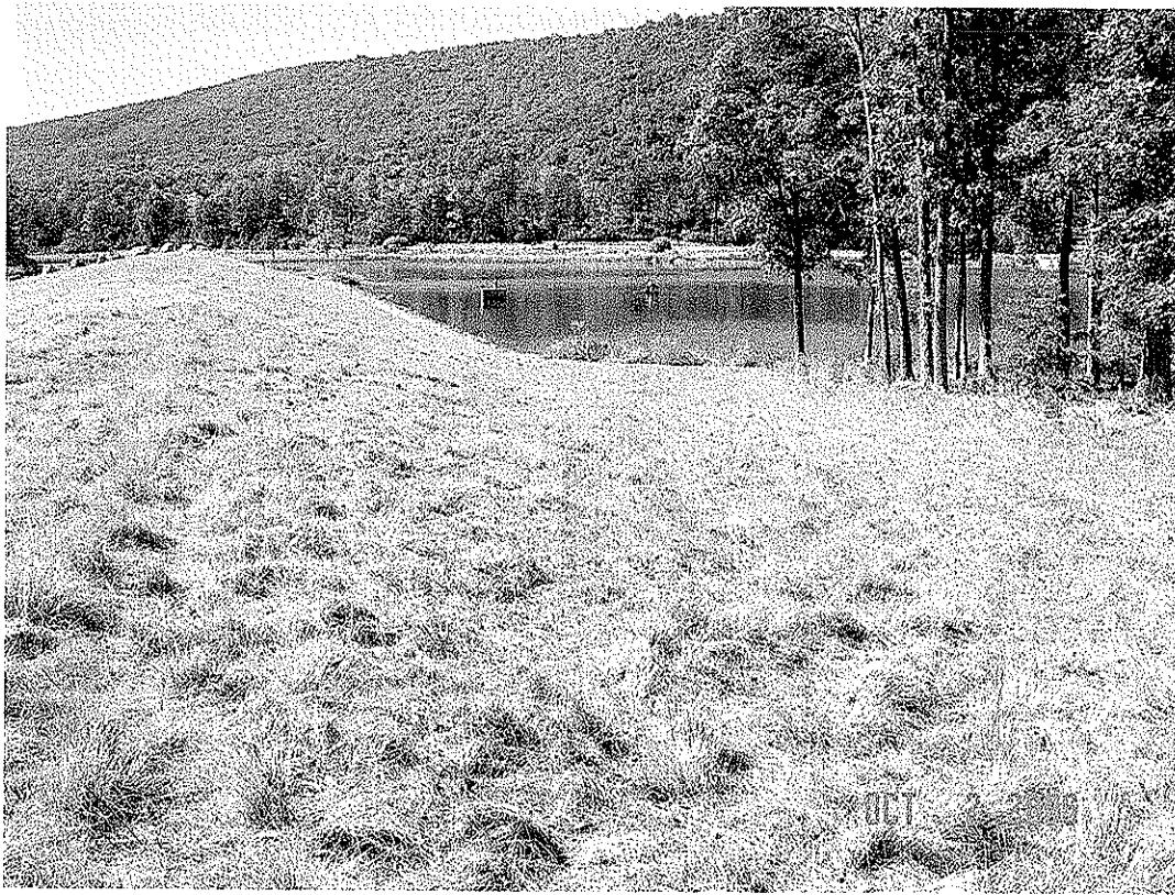
WARDEN LAKE DAM MODIFICATION, HARDY CO., WV
