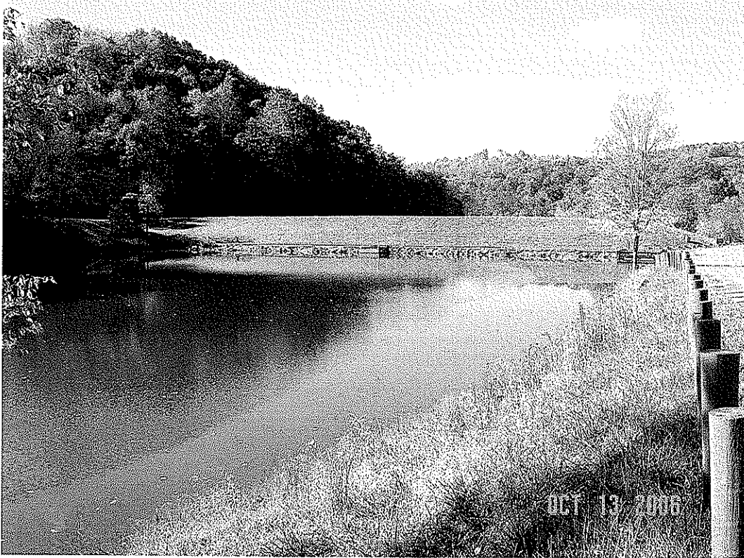
JIMMY LEWIS DAM MODIFICATION, MERCER CO., WV
