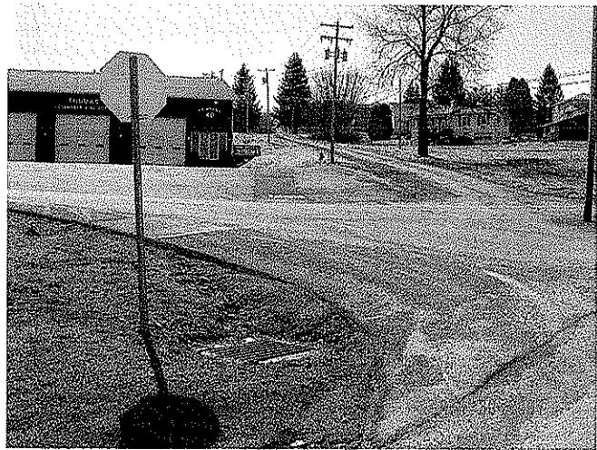
New Storm Drains and Catch Basins
