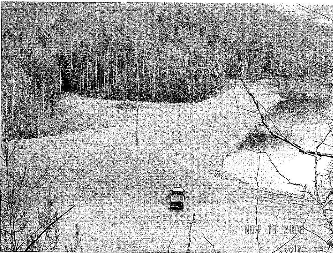
PLUM ORCHARD DAM MODIFICATION, FAYETTE CO., WV
