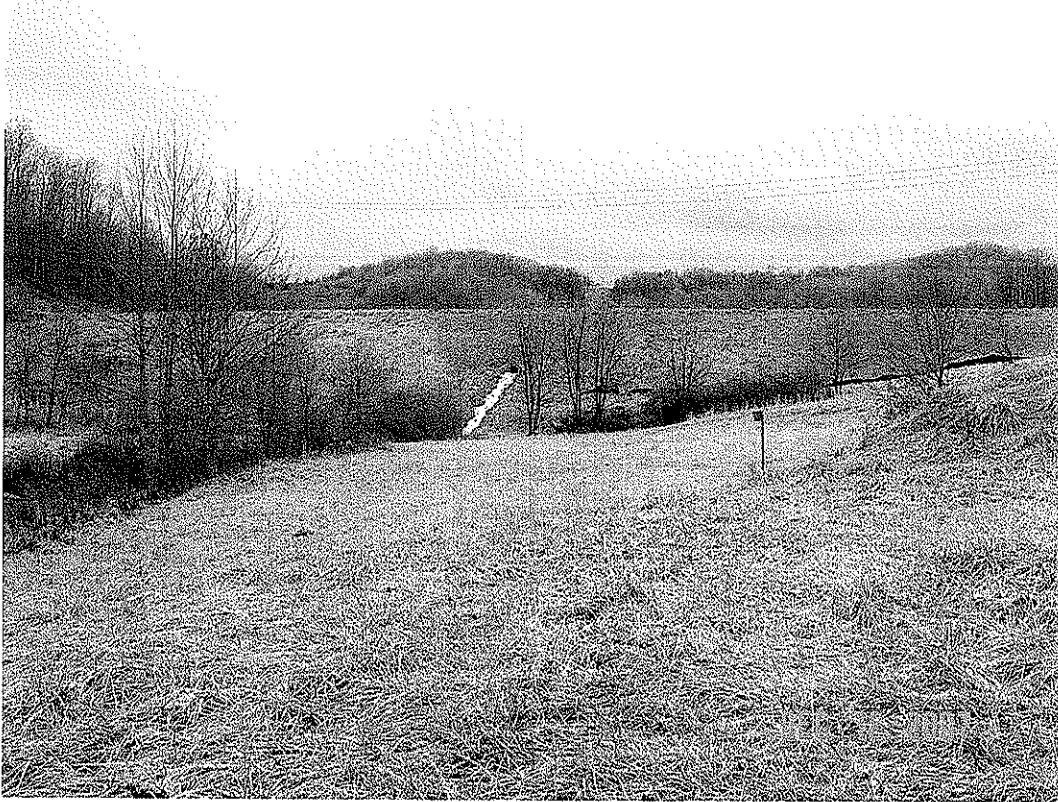
LEMLEY DAM MODIFICATION, MONONGALIA CO., WV
