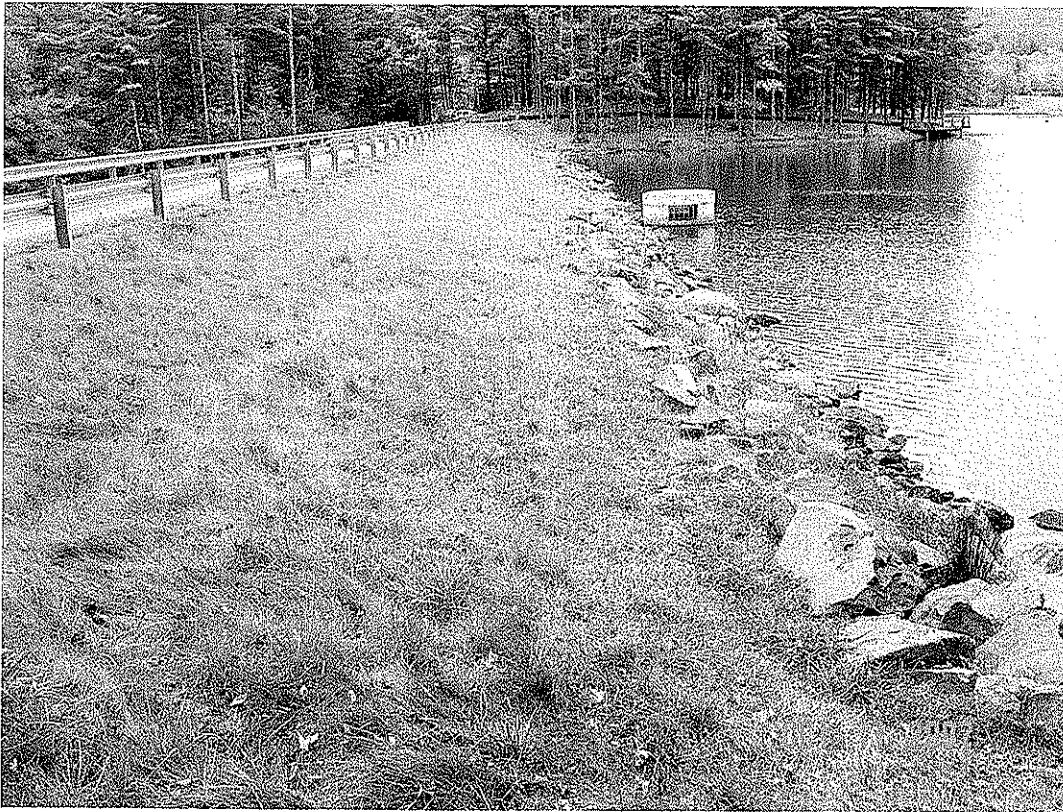
MONCOVE DAM MODIFICATION, MONROE CO., WV
