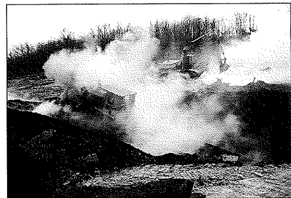
Jamison Burning Refuse Reclamation Project
