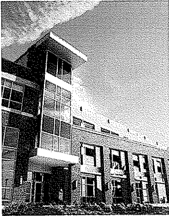
WVU Transportation Center & Garage
