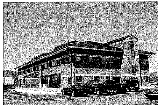
WVDOH D-6 Office Building, Moundsville, WV
