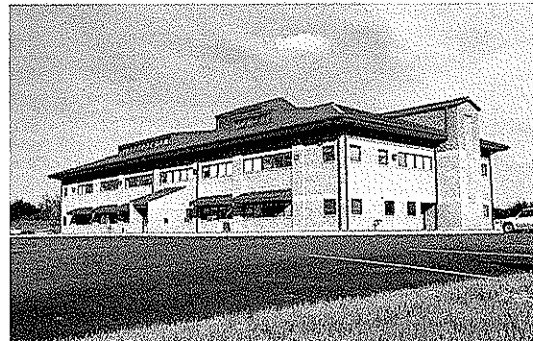
WVDOH D-10 Office Building, Gardner, WV
