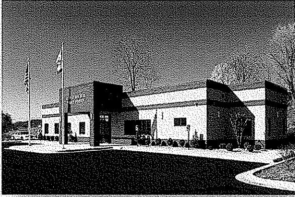
The City of Oak Hill's new Police Station was a publicly funded project completed on time and within budget in the summer of 2009
