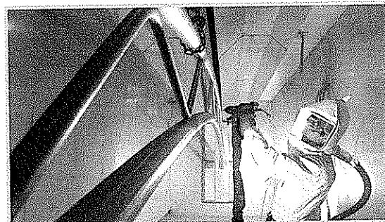
Molten Zinc Protection Process
