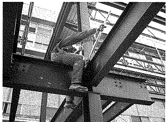
Thrasher Engineering provides various materials testing and inspection services for the expansion of West Virginia University's Ruby Memorial Hospital and the addition of the Health Science Learning Center.
