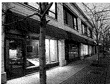
BOSTWICK DESIGN PARTNERSHIP OFFICE BUILDING HISTORIC MIDTOWN DISTRICT CLEVELAND, OHIO
