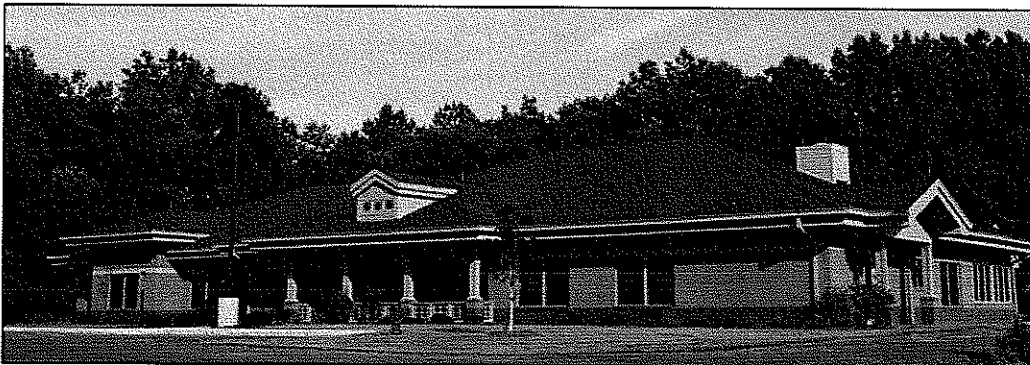
Transitional Facility at William R. Sharpe Jr. Hospital
