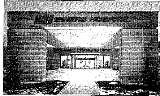
Miners Hospital of Northern Cambria. This new, modern facility, completed in September 1999, replaced Northern Cambria County's 30-year-old hospital.
