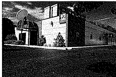
The renovations and expansion of the WBOY offices required a roof replacement
