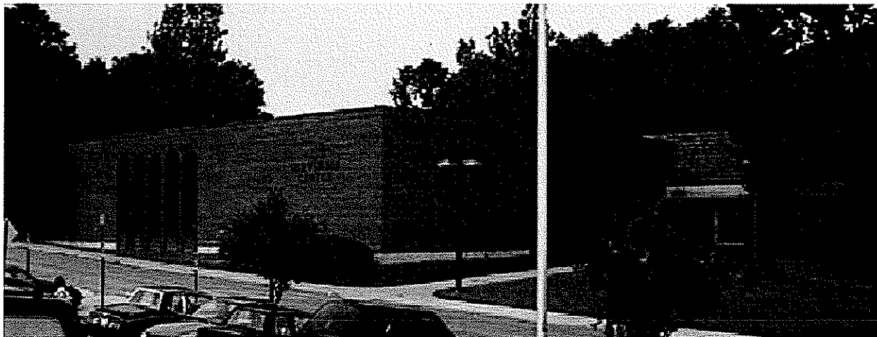
Stevenson Library – Renovations
