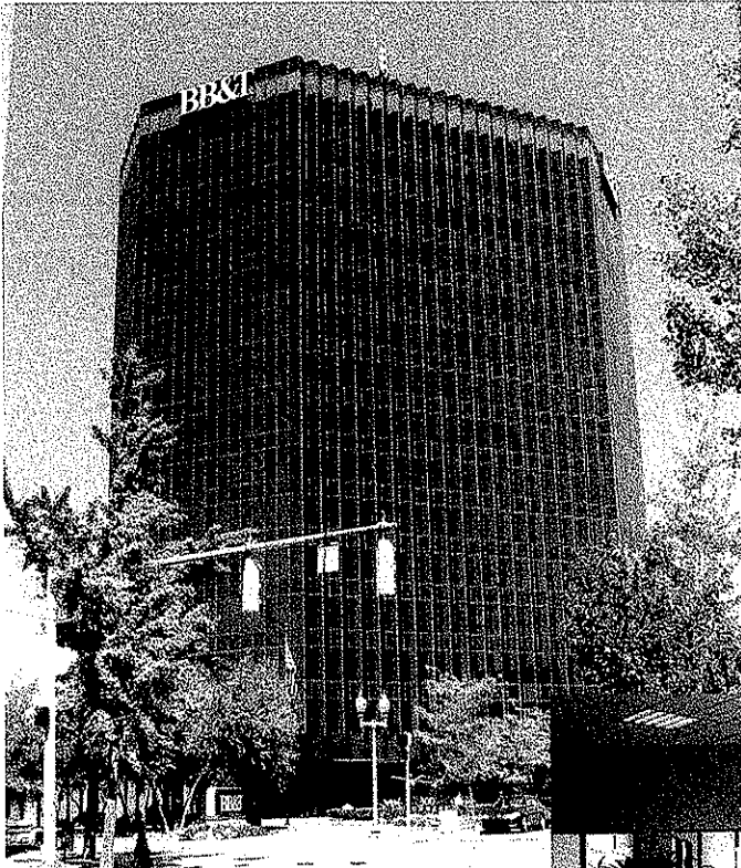
Multiple Tenant Build-Outs and Lobby Renovations Branch Banking & Trust
