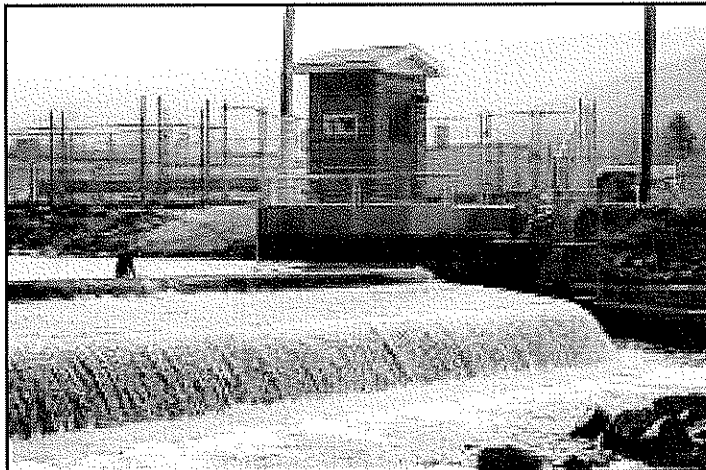
Rebuilt Water Intake Structure
